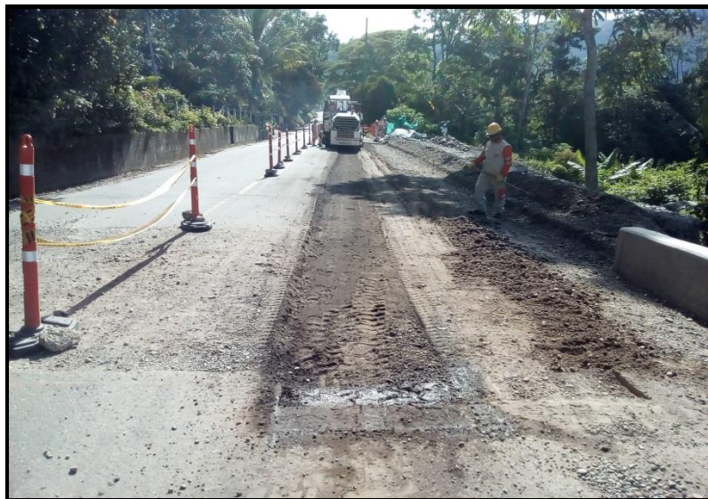
FRESANDO PR37+902.5 AL PR 37+943-DER
